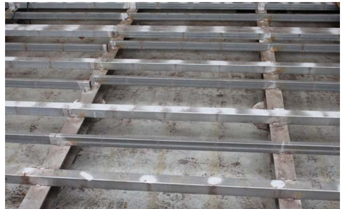
Figure 28: Method 2 - Knee Bracing At Beam - Post Locations
