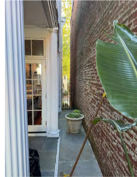
View of existing side yard from rear yard (facing east).
