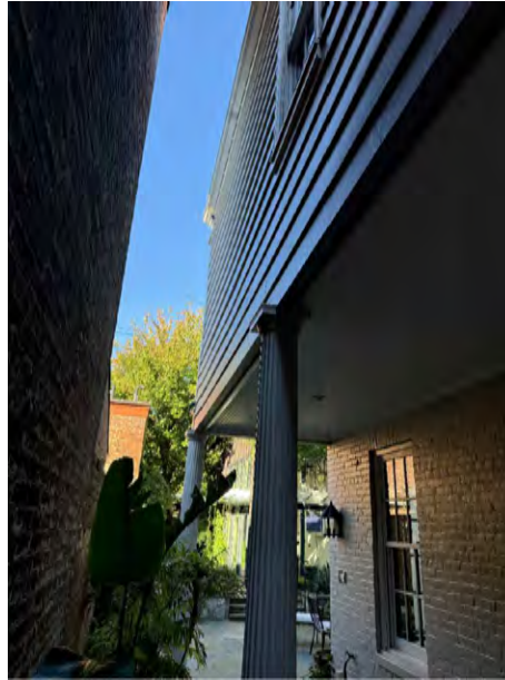
View of existing building where infill at First Floor is proposed.
