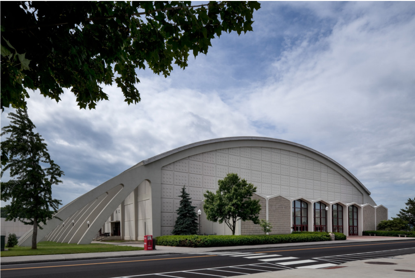
1964 - Cassell Coliseum; Free-Spanning Concrete and Laminated Wood Dome
