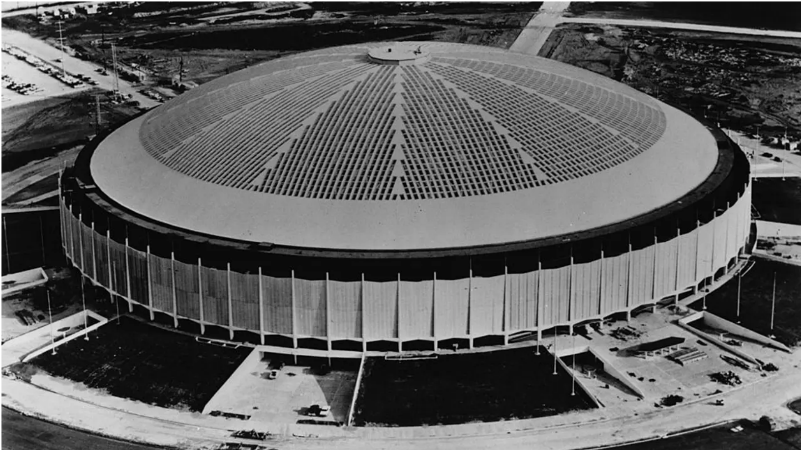
1964 - Houston Astrodome; Steel Lamella Dome
