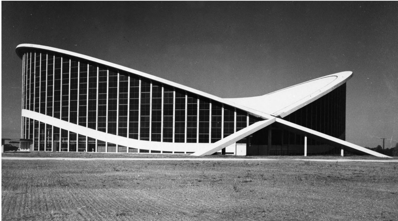
1952 - Dorton Arena; Hyperbolic Paraboloid Dome
