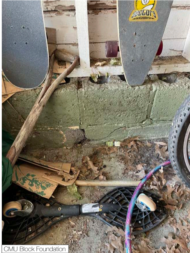
CMU Block Foundation
